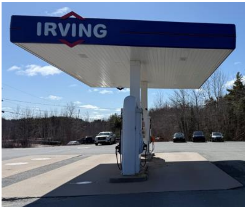
Gas pumps and canopy
