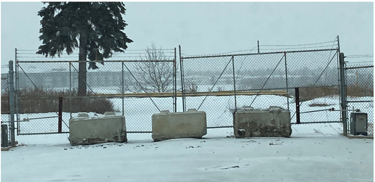
West Gate Secured with the Jersey Barriers
