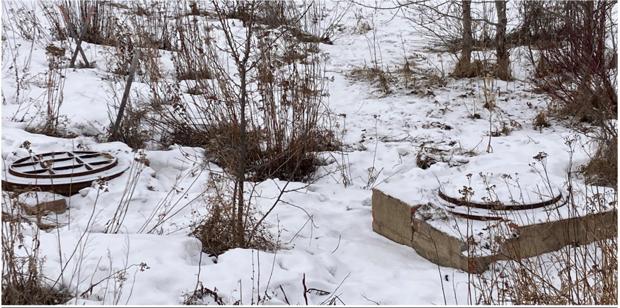
2 of the 9 Manholes Welded Up to the Electrophone Corridors
