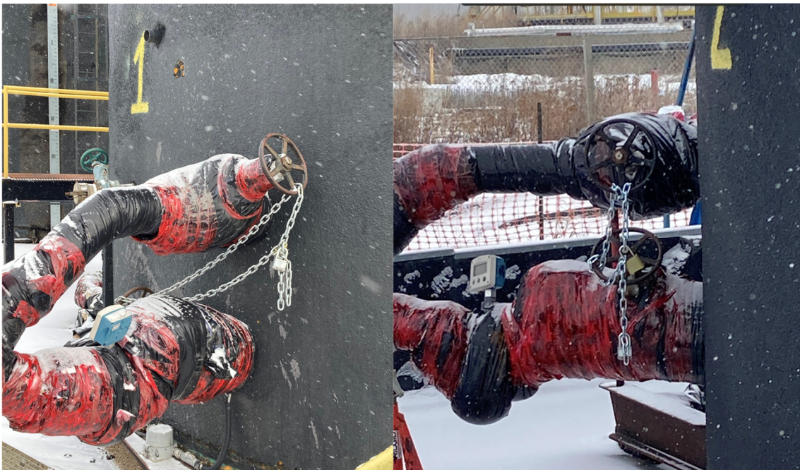
11-17-53-23 W4 Tanks 1 & 2 Cleaned Out and Secured
