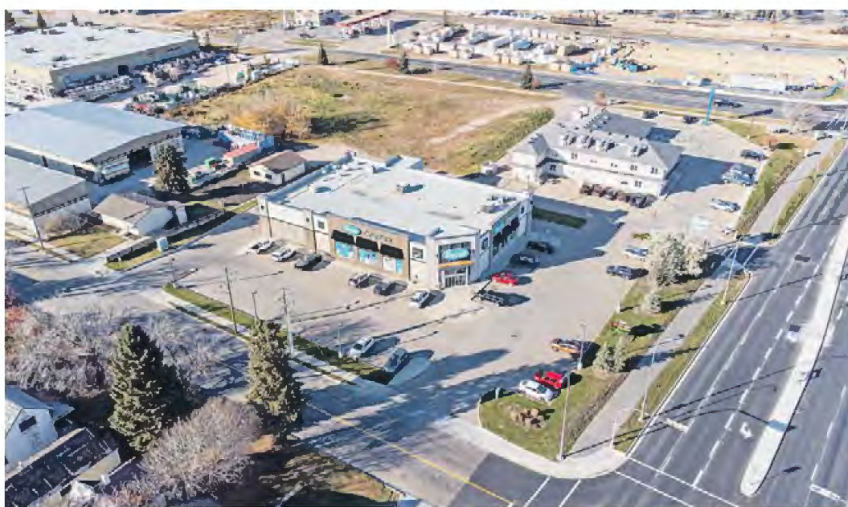
A Rexall-occupied building in Stony Plain, Alta., was recently purchased by a B.C.-based private investor. The total number of ‘smaller commercial real estate’ transactions in Canada in 2021 is expected to reach 9,500, according to CBRE, which would surpass the previous record by 2,000 transactions.
